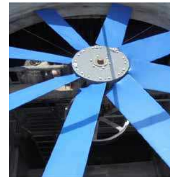
Replacing the aluminum fan blade to FRP energy conservation fan blade in the cooling tower
