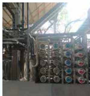
EPI waste water recycling system
