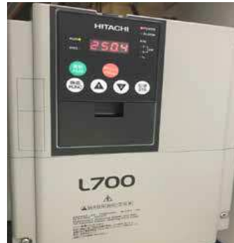
Using new type of ASM fan frequency converter
