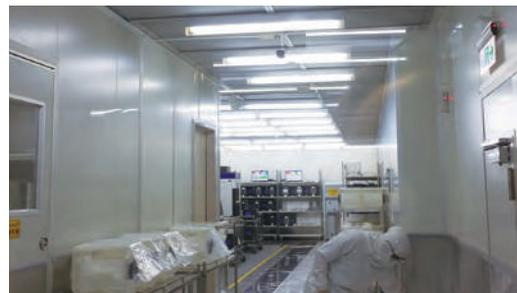
Traditional Light Tube Replaced by LED High Efficiency Light Tube
