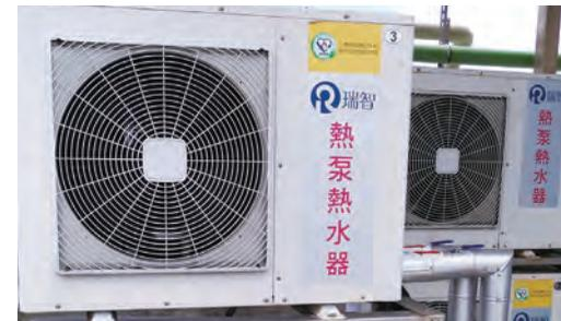
Diesel Water Heater Replaced by Heat Pump Water Heater + Electric Water Heater
