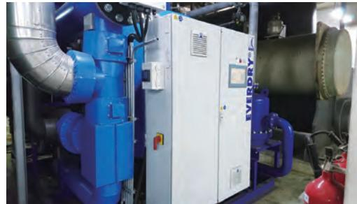
Heat of Compression Air Dry Added to Replace Existing Heated Desiccant Compressed Air Dryer
